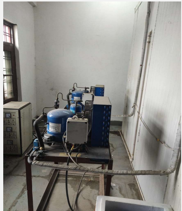
Fig 4: Condensing Unit for WIC
